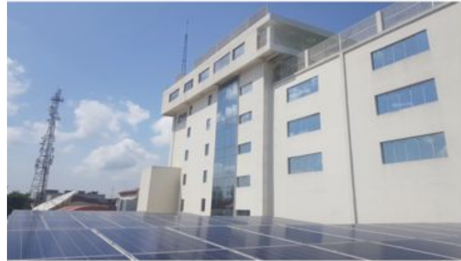
21st Century Datacenter in Lagos (Nigeria)
